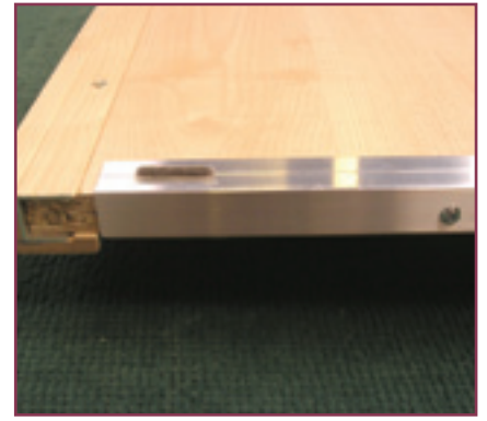
15. Attach the top aluminium rail by using your 3mm drill bit and dome head screws through the aluminium rail into the TOP edge of your panel in two positions equally spaced. Turn the panel over and lay it flat on it's back. The batons are no longer needed.
