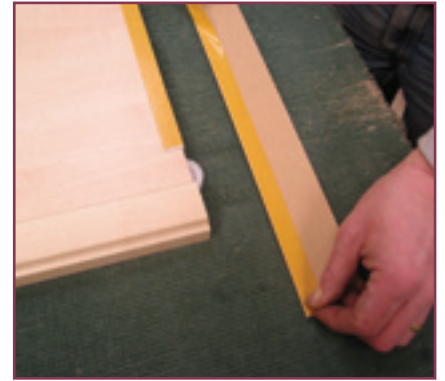
18. Apply a length of double sided adhesive tape to the back, top edge of the 55mm bottom trim.
