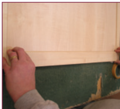
20. Attach the 55mm trim, applying plenty of pressure.
