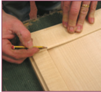
17. Mark the width of the 55mm trim with a pencil about 2mm wider than necessary. (This will allow a tight fit when you are ready to fix)
