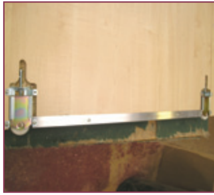
14. Repeat the other side and complete by adding two screws equally spaced along the aluminium rail into the BACK of the panel.
