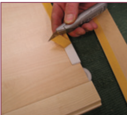
19. Remove the yellow part of the double-sided tape of the 55mm trim and the bottom aluminium rail.
